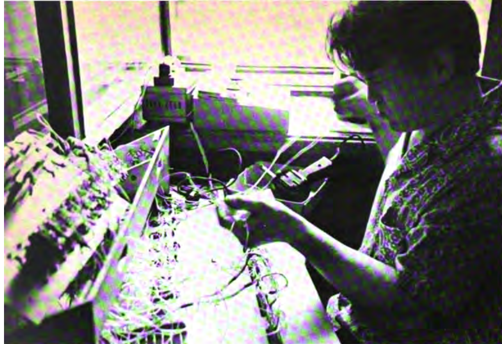
Sergei Sirotkin, one of the four blind-deaf Moscow University students, repairing a teletactor, a machine that converts the click of a typewriter key into a pricking felt by the fingertips. Different combinations of the prickly sensation denote different letters.
