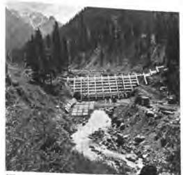
These structures not only protect the valleys from mud floods but change the topography in the area, making slopes less steep. Damming is a most effective guard against flooding by mud.
