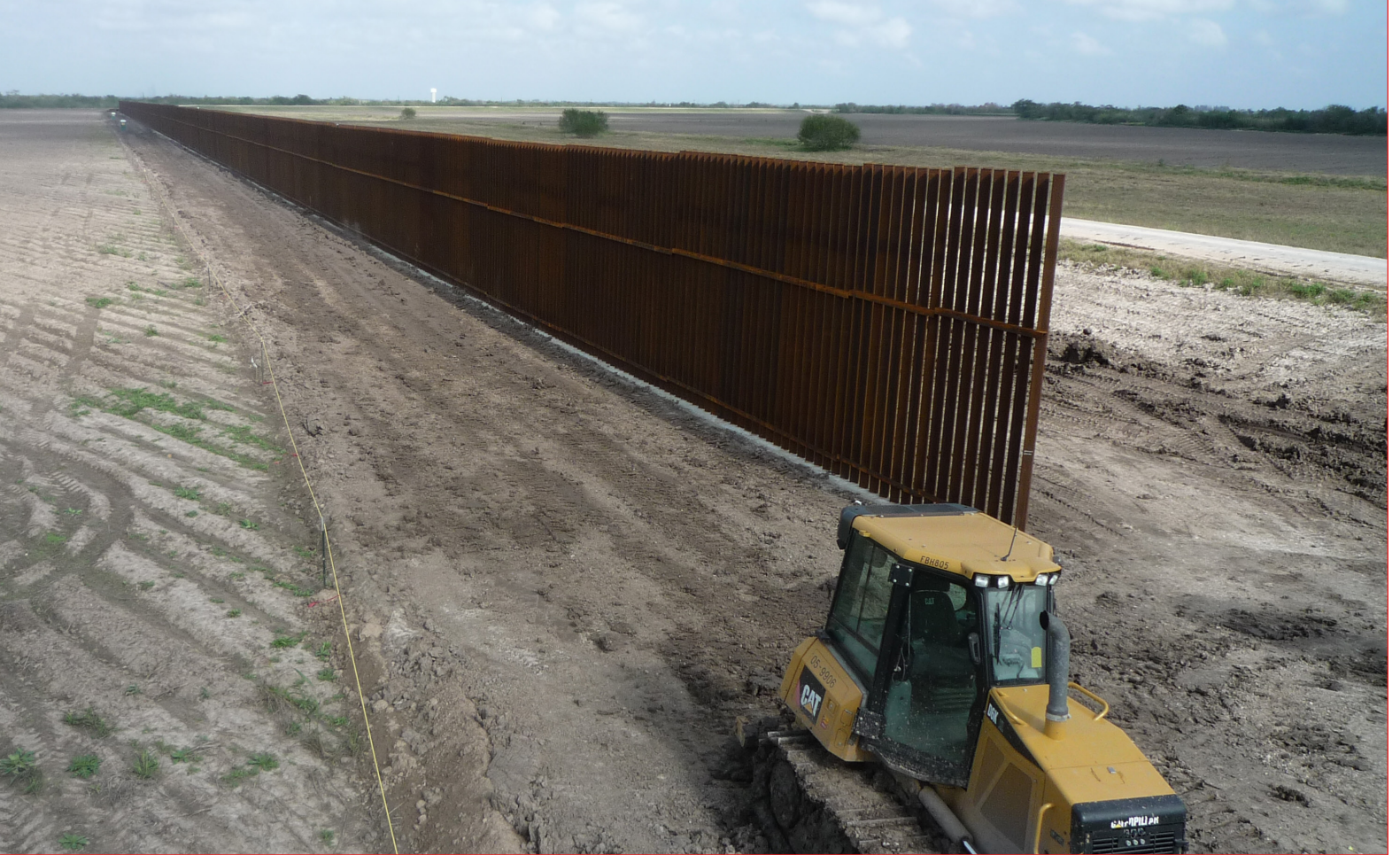
Construction of the US-Mexico border fence
