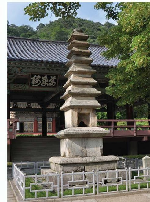
The rectangular nine-storeyed pagoda in the architectural style of the early Koryo period, is 6m tall. It was erected in 1044, according to the record carved on the back of the first storey of the body.
