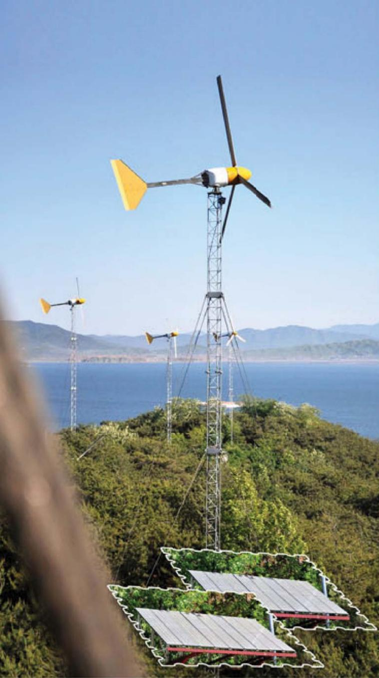
Windmills and solar panels produce electricity for the management of the dockyard
