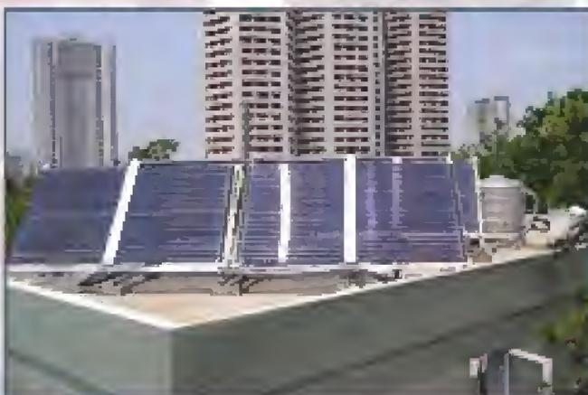
These solar water heaters are designed to heat water up to 45° C in summer, 70° C in autumn and 50° C in winter.
