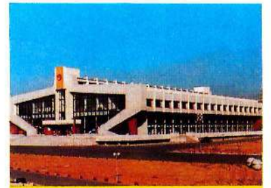
Indoor Swimming Pool Complex
