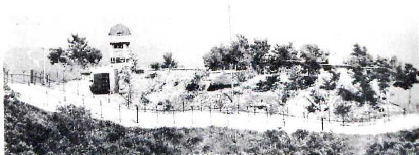
Part of the concrete wall
