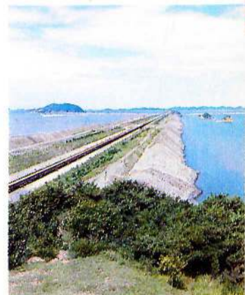
A long-distance belt conveyor makes land wider
