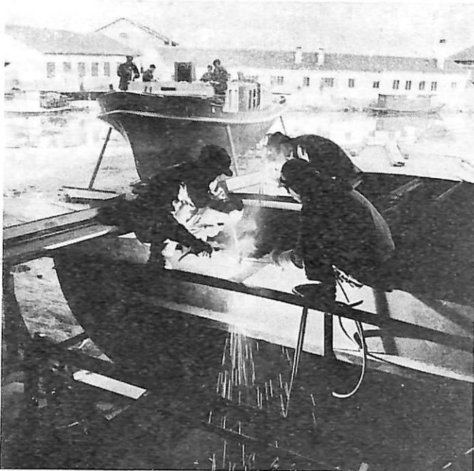
Welding the hull of a motorboat in Chienchow commune's shipyard.
