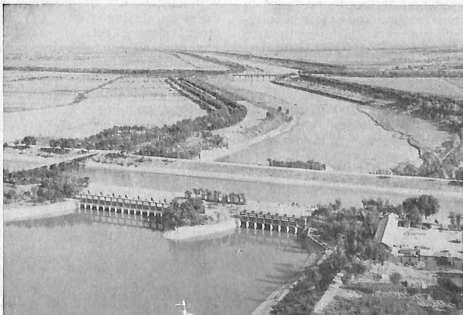
A newly completed siphon station, one of many water conservation works that control floods and waterlogging in the Haiho River basin.
