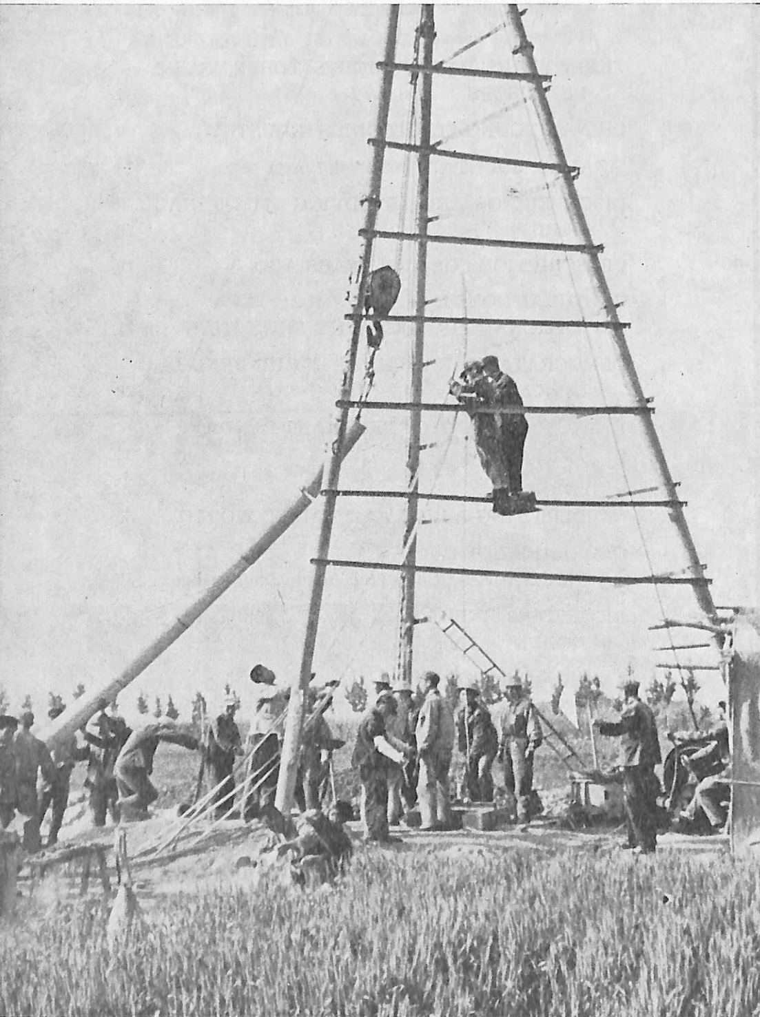
Well-drilling team of Wuchiang county, Hopei province, taps underground water for a commune.
