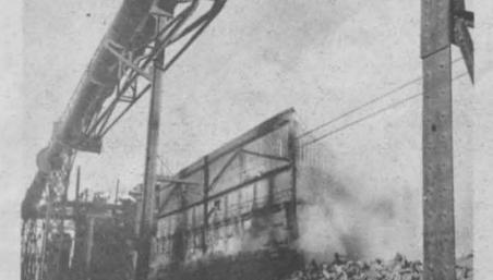
Hot coke from the ovens is cooled by water before passing to the next process
