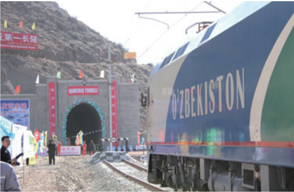
A train stops at the entrance to the 19.2-km long Qamchiq Tunnel in Uzbekistan, which is completed on February 27, 2016, as part of the China-Kyrgyzstan-Uzbekistan Railway
