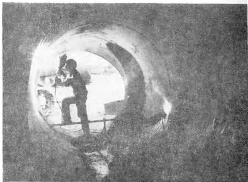
Welding a water pipe at the Pha Lai thermo-power plant built with Soviet assistance.
