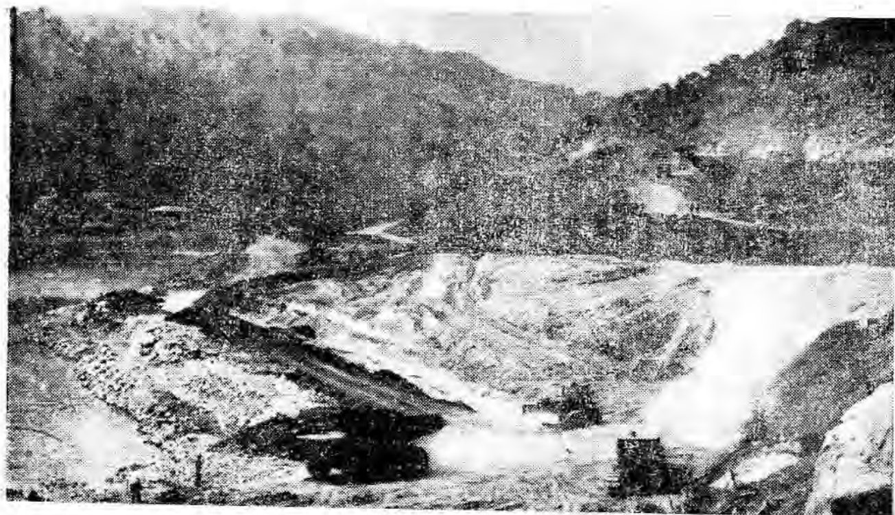
Partial view of the construction site of Da hydro-electric power plant.
