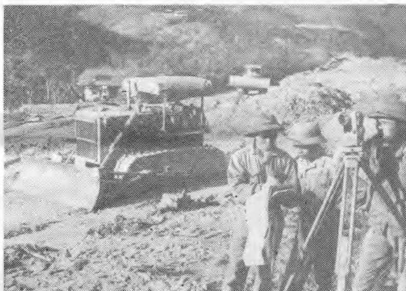
Building roads for the dam on the Da river.
