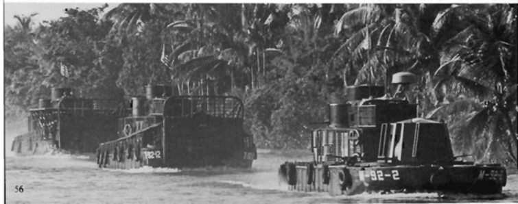
The differences between an ATC and Monitor can be seen here. The most evident difference is the spoon bow of the Monitor mounting a 40mm turret. (US Navy)
