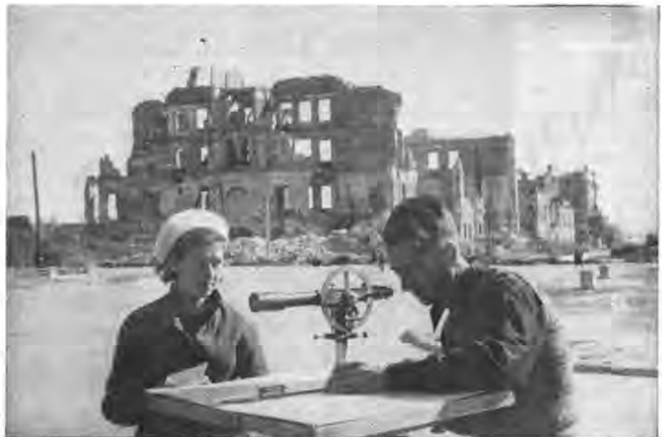
Surveyors measure the streets of Stalingrad. Plans have been made for construction of new squares and residential sections in the completely gutted city
