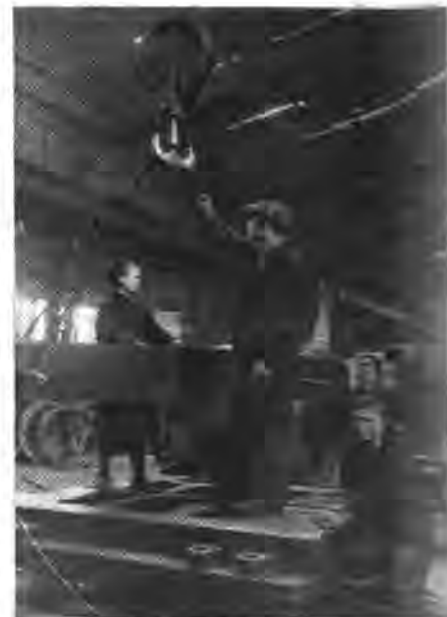
A Leningrad plant which produces electrical equipment
