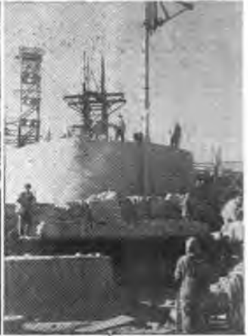
Work starts on a 350-foot smokestack at Orsk-Khalilov coke-chemical plant
