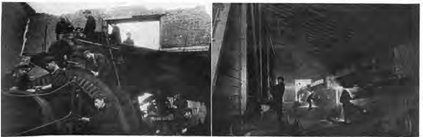
RESTORATION—Inhabitants of Orel restoring the Diesel in their city's electric power station; (right) one of the restored shops of the Kalinin train-car building works
