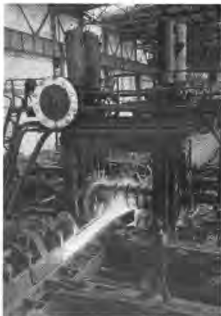
Rolling steel pigs through the cylinders of a blooming mill at the Stalin metallurgical works in Magnitogorsk
