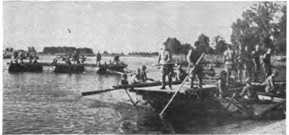
Soviet sappers build a pontoon bridge over the Narew River
