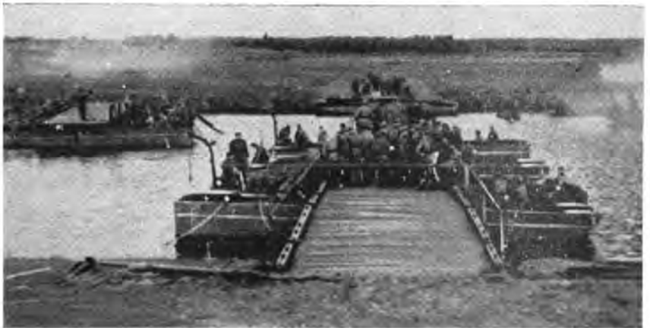
Connecting up the separate sections of the bridge across the Narew
