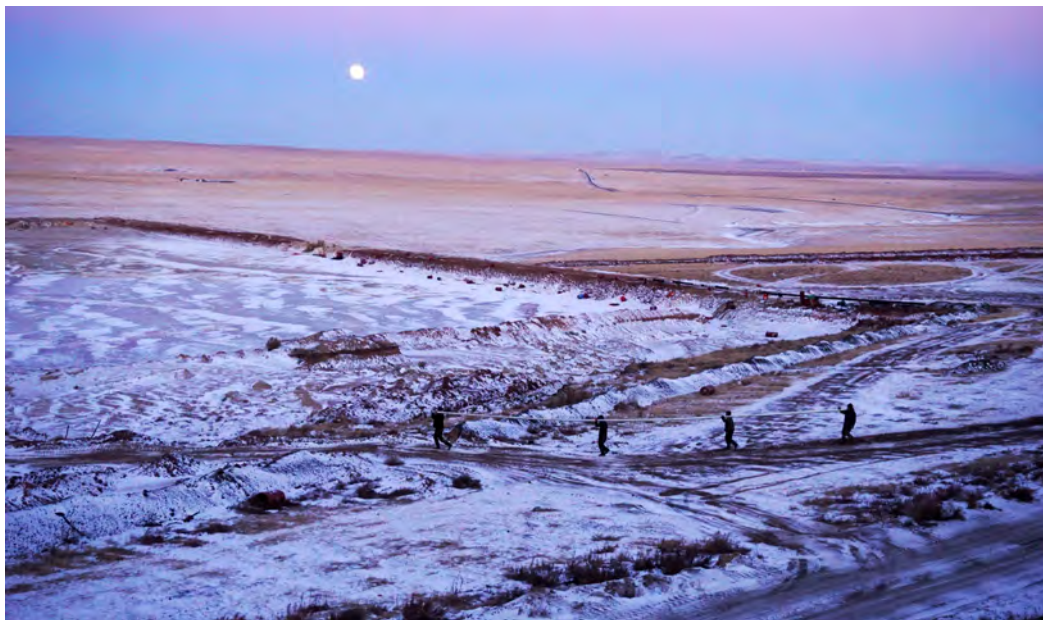
Four workers carry an insulated water pipe across the snow-covered grounds of the mine.
