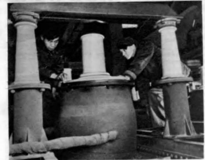
Workers of the Mukden Metallurgical Works maintain the efficiency of the electric dust collectors by constant overhauling. Smoke and dust contain many valuable materials which can be collected and refined
