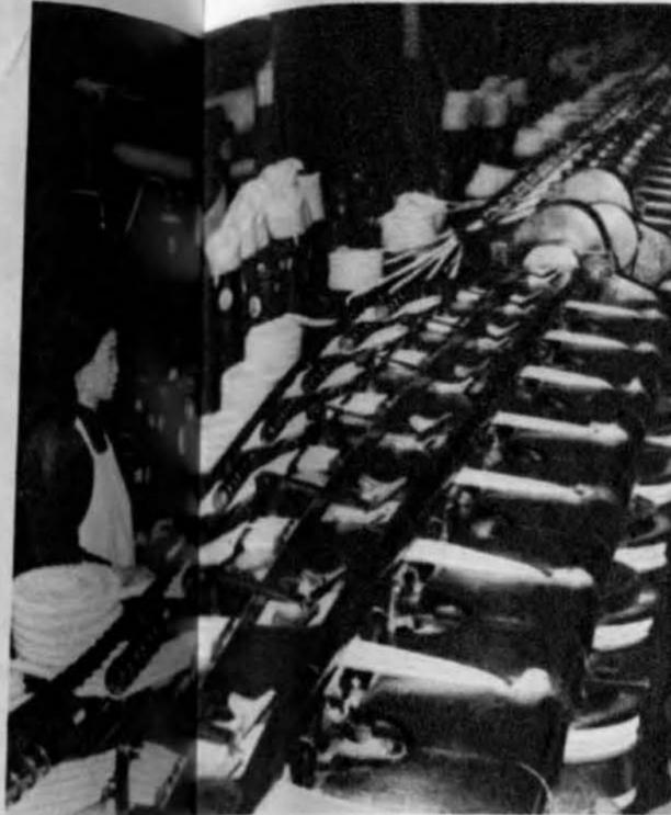
**SLUBBING**—slivers run through a slubbing or roving frame and are twisted and drawn to an even thickness. This drawing slues irregularities in the thickness of the slivers
