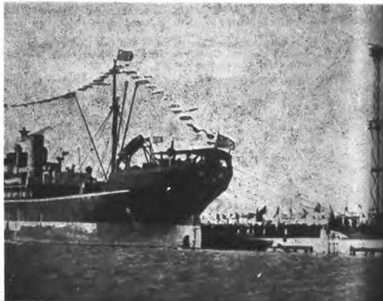
The 10,000-ton S.S. 'Changchun' anchored at the No. 1 pier of Tangku Harbor when the harbor was officially opened last October.
