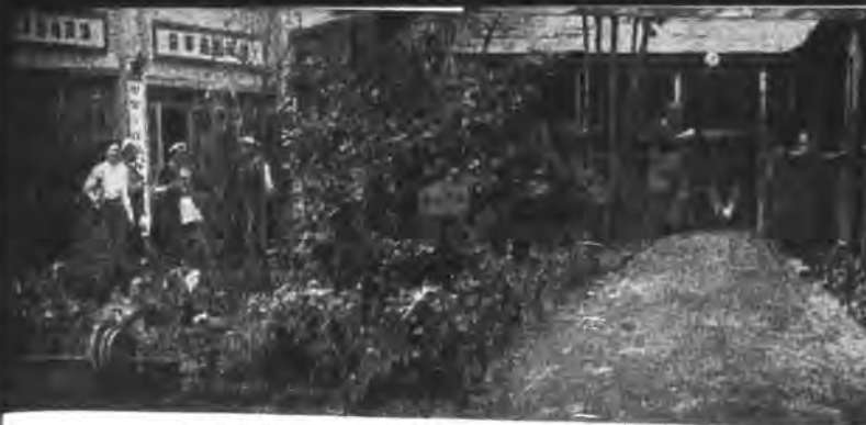
A clubhouse built by transport workers of the Huashun Wharf in Shanghai from scrap materials.
