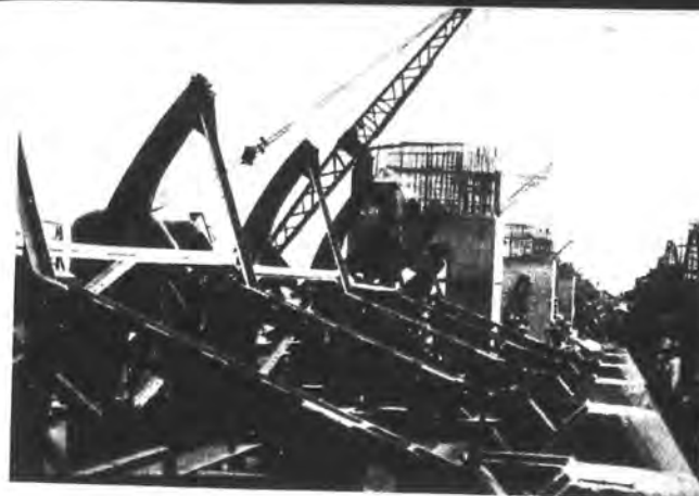
A section of the one kilometer-long Tapingkuo sluice gate at the upper end of the basin.
