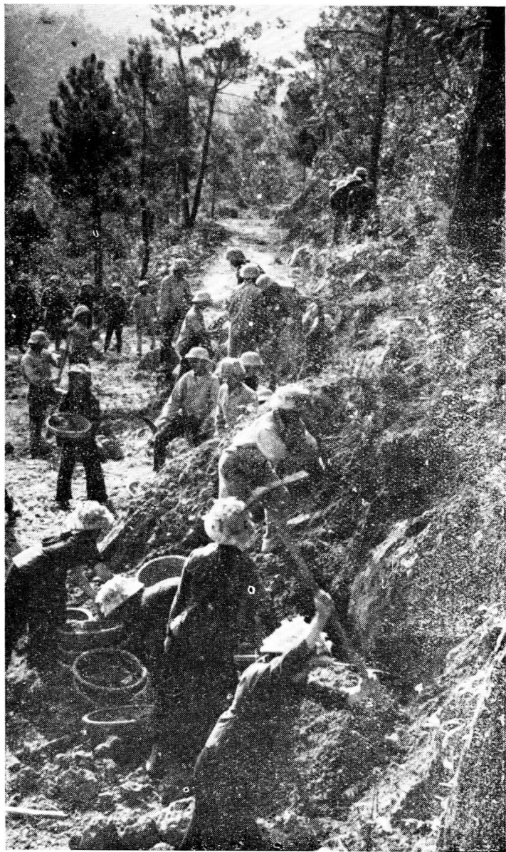
Repairing bombed roads.
