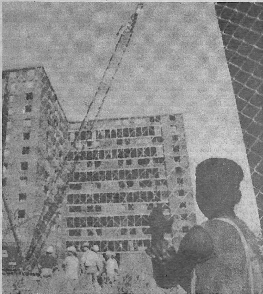
Demolition of a public housing project building in Chicago.
