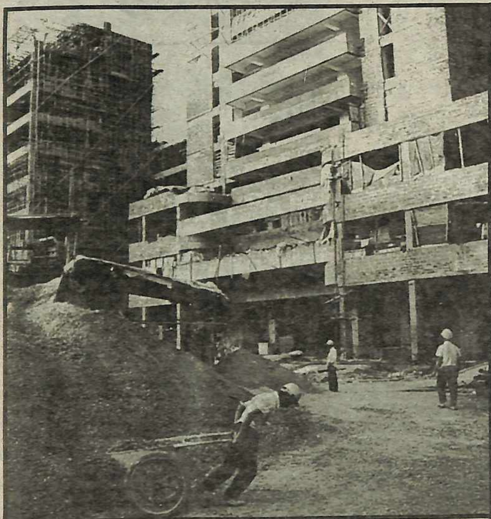
Construction site in Haikou.
