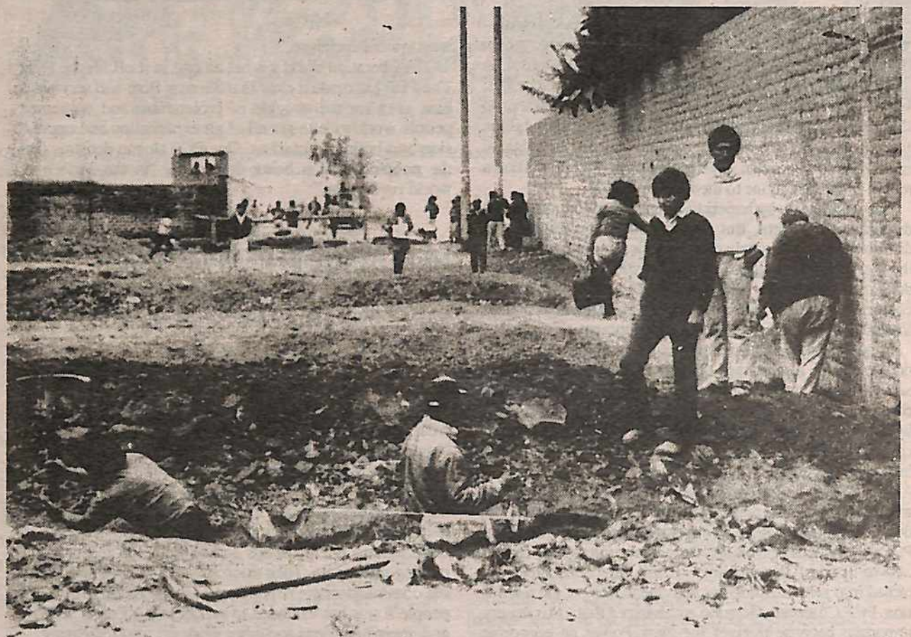
Raucana residents dig trenches to block police assault.
