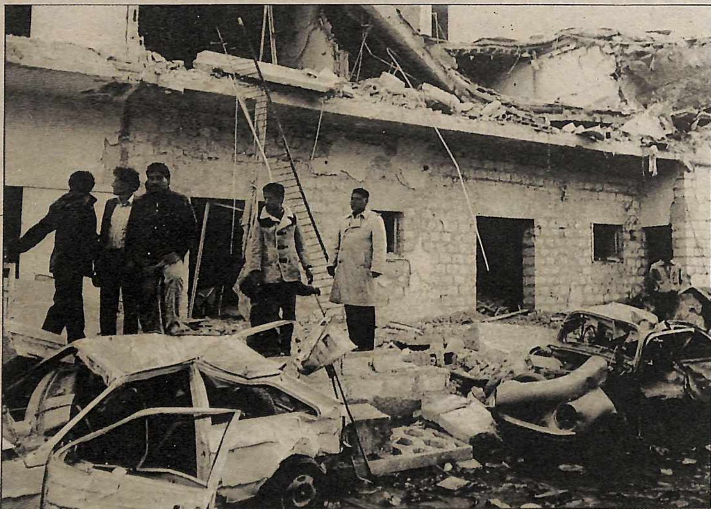
Damage by U.S. bombs in Libya, 1986.
