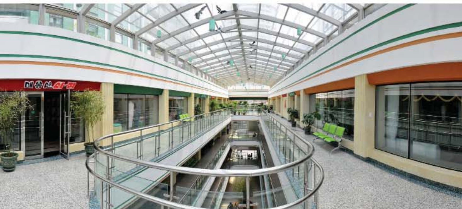
General commercial outlet furnished on the ground floors linking the 70-storey skyscraper with the 55-storey one
