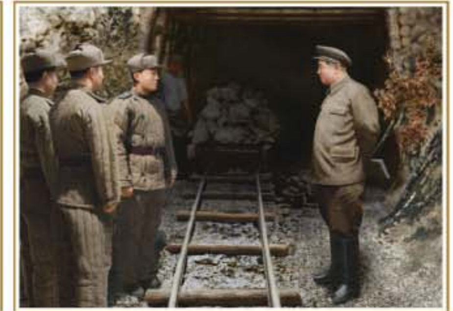
Kim Il Sung inspects the tunnelling site [October Juche 40 (1951)].
