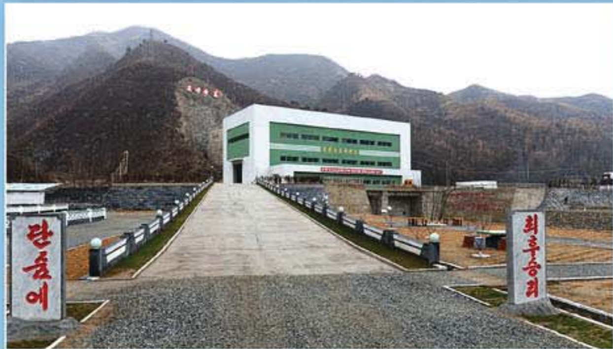
Huichon Power Station No. 3
