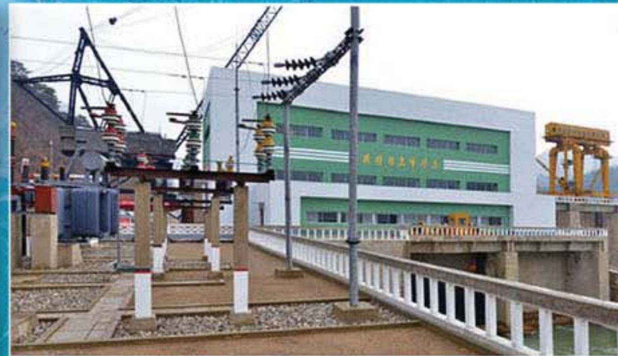
Huichon Power Station No. 8
