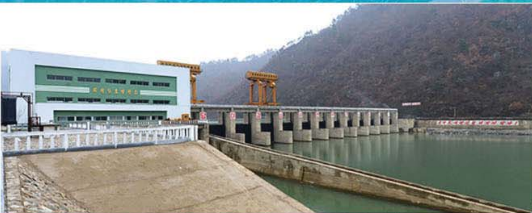
Huichon Power Station No. 9
