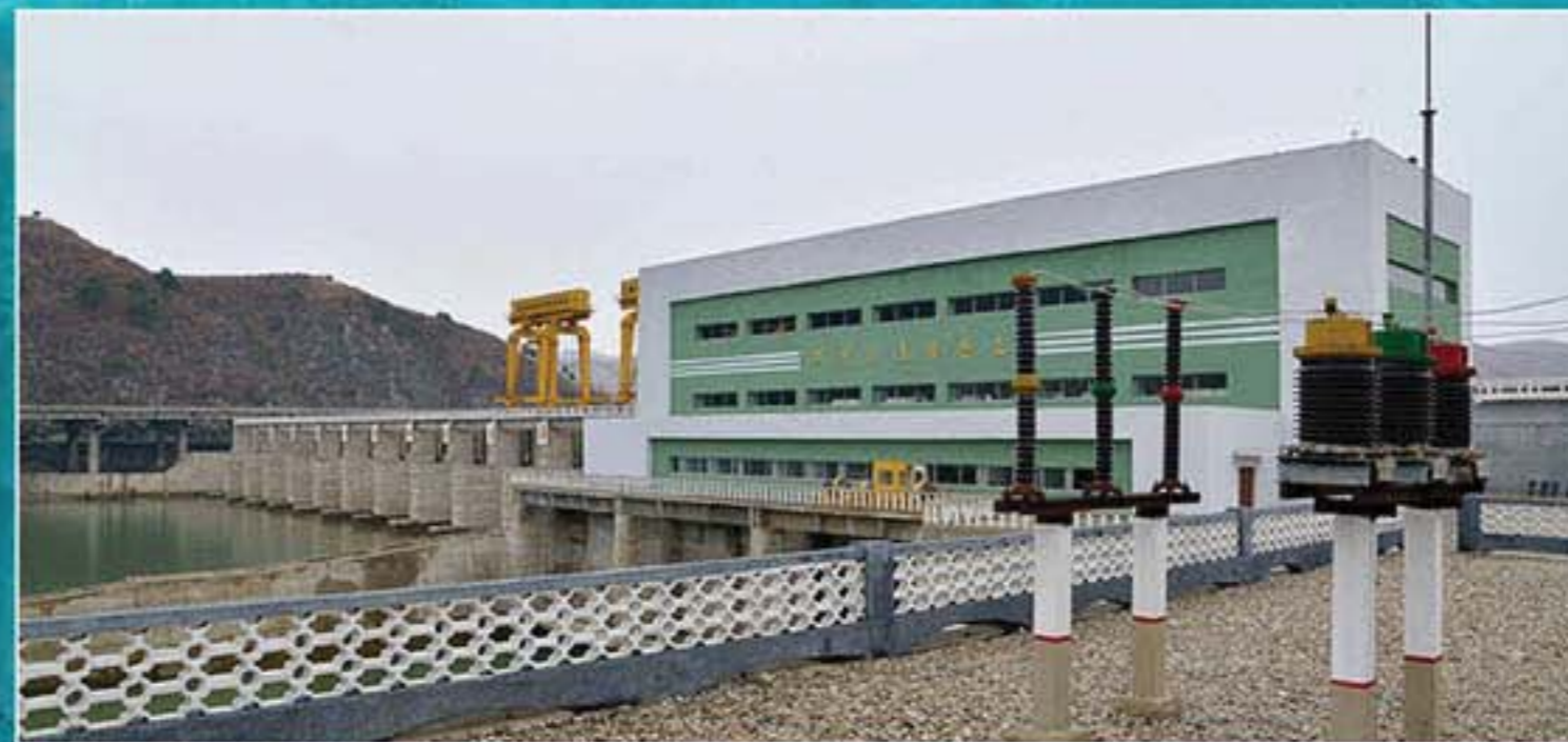
Huichon Power Station No. 11
