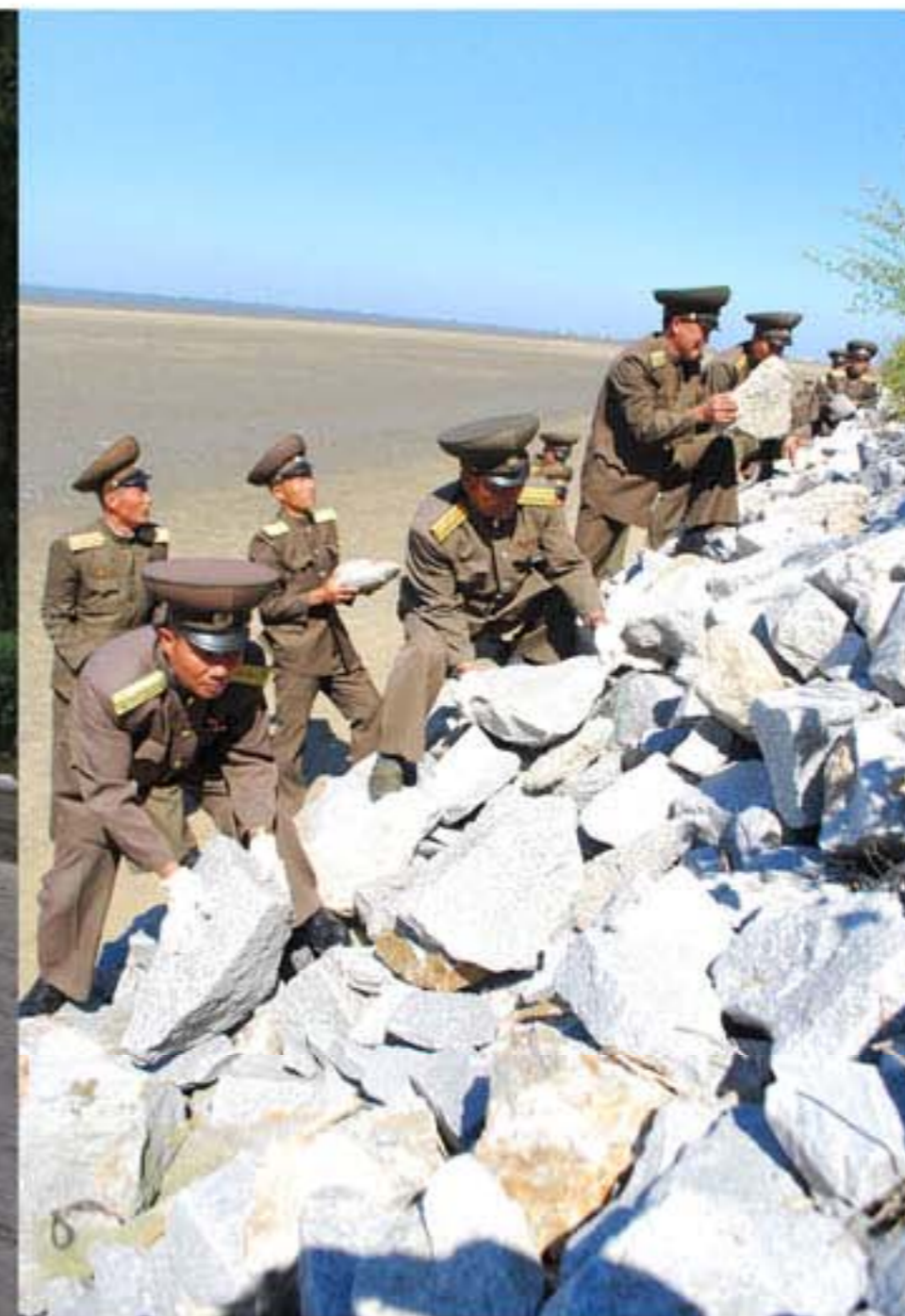
They are regularly reinforcing the coastal embankments
