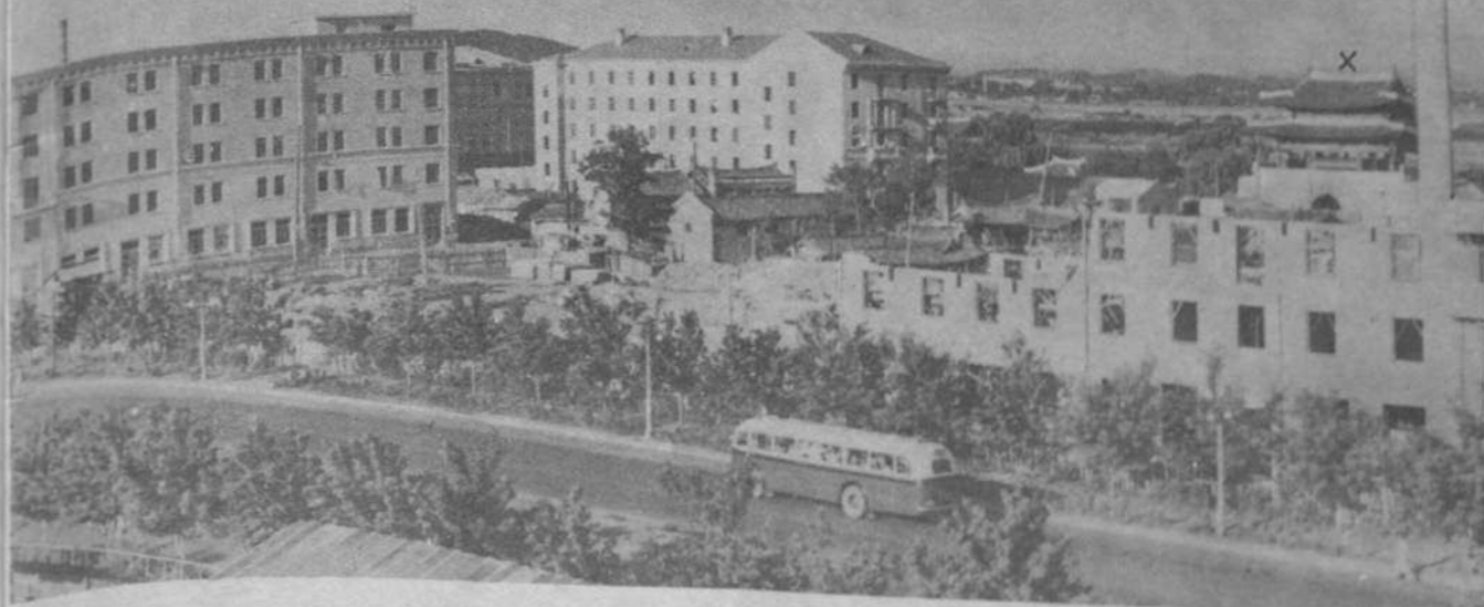
Present-day Taidong-moon Street under reconstruction (X in the center denotes the Taidong-moon Gate)
