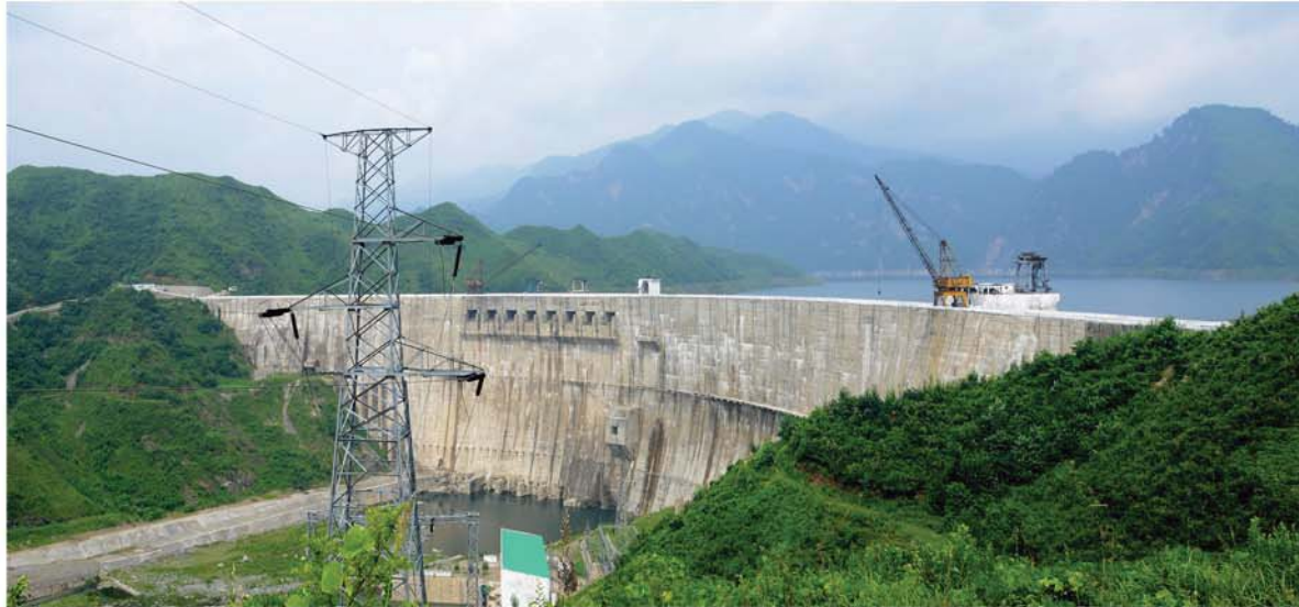
The Kumyagang Army-People Power Station.
