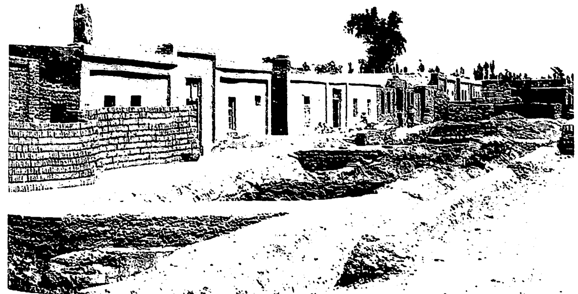
New buildings constructed by the second production brigade of the Burning Mountains People's Commune
