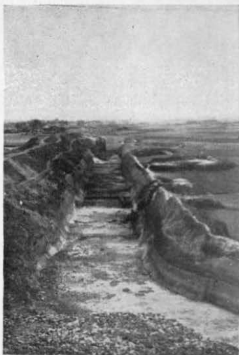
A GOVERNMENT TRENCH.
