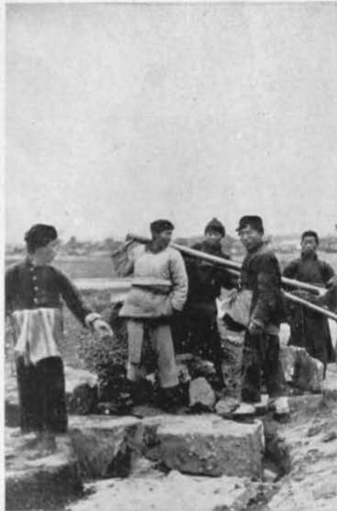
LAYING FOUNDATION OF BLOCKHOUSE.
