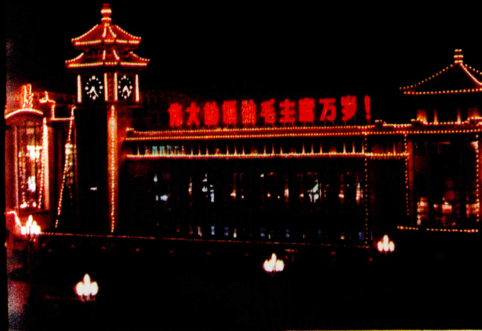
The Peking Railway Station at night.
