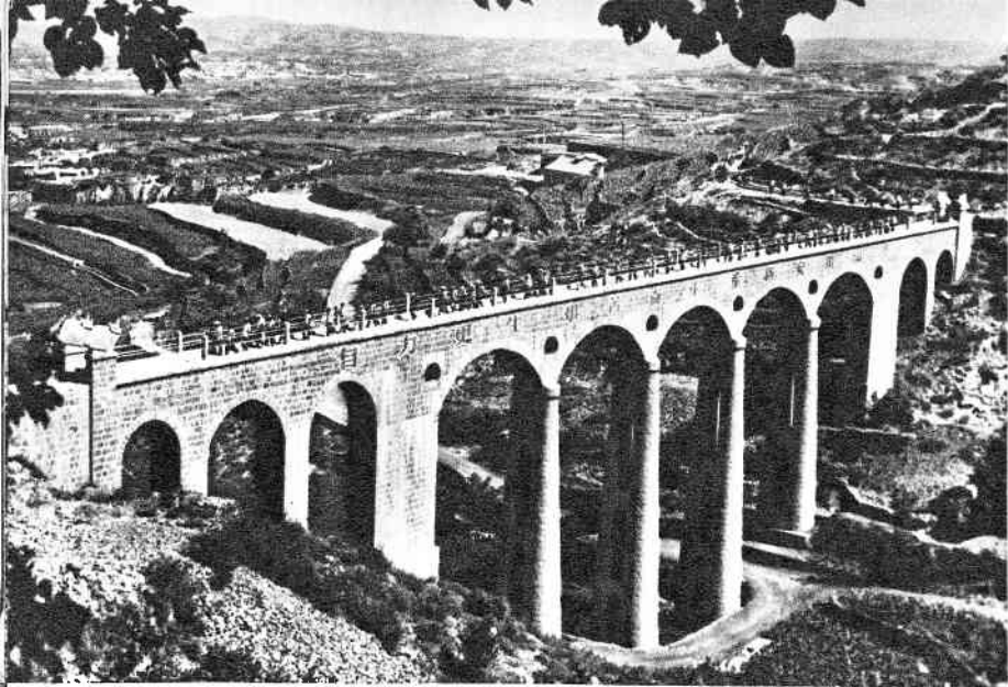
Unity Aqueduct, built in 1974.
