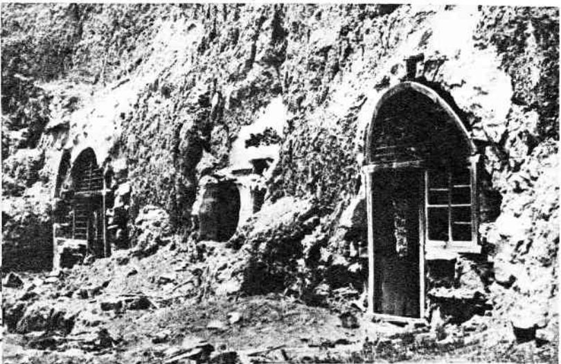
Many cave-dwellings in Tachai collapsed in the big flood (below). Soon afterwards, the Tachai people built their new housing by self-reliant hard work (above).
