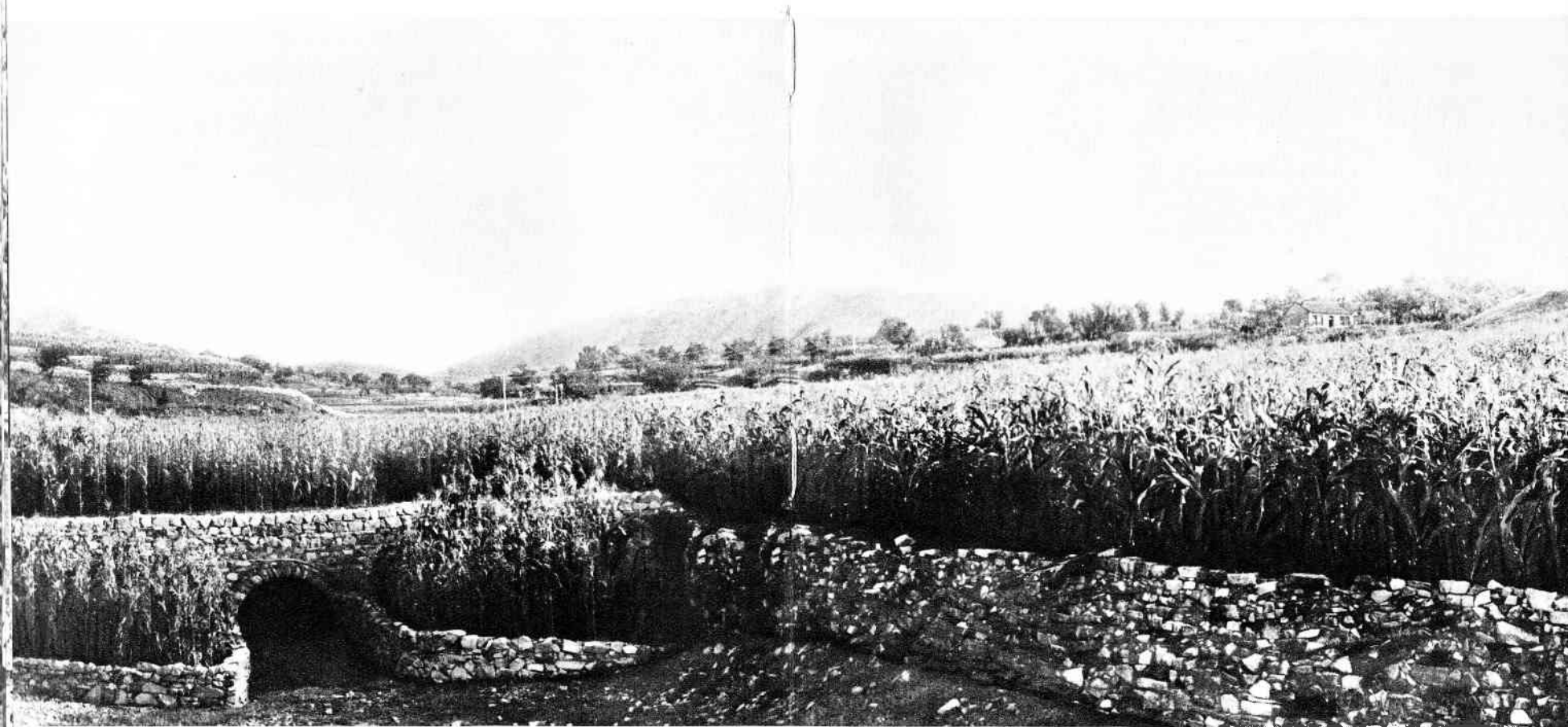
The former rock-bound East Gully has become a granary.
