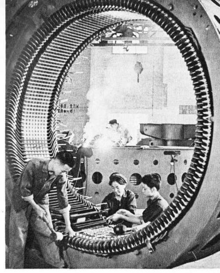
Chinchengkiang, a small town in the mountains of the Kwangsi Chuang Autonomous Region, now makes 3,200-kw. water-turbine generators.
