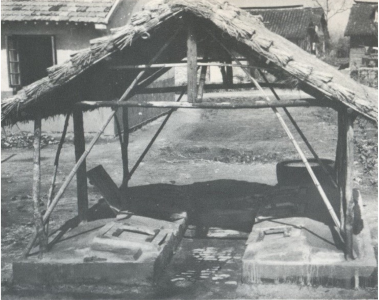
...One of the hygienic village latrines which they constructed.
