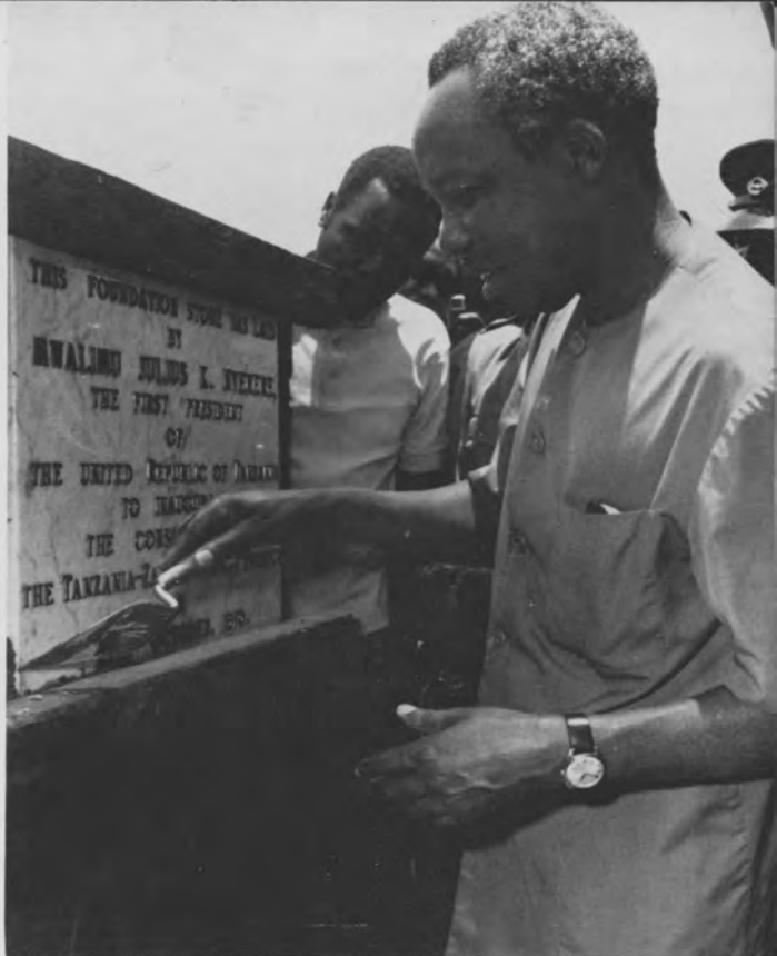
4 President Nyerere laying the foundation stone of the Tanzam railway on 28 October 1970 at the Zambian terminal of Kapiri Mposhi.
