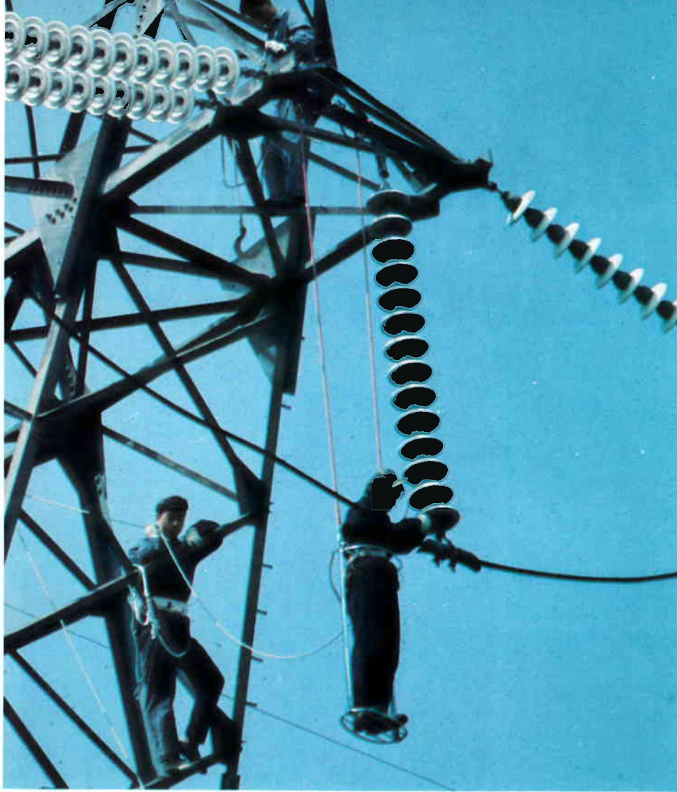
Live-line electrical workers help bring "power to the people." (Photo: D. Cox)
