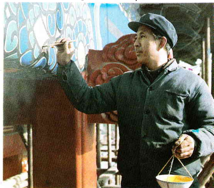
Restoring old painted designs in a delicate operation.
