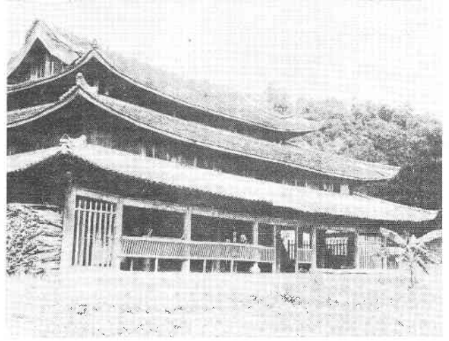
In Menglian county, a sweep of multi-tiered roofs graces the former headquarters of the despotic local headmen who for centuries ruled the area. Xie Jun
