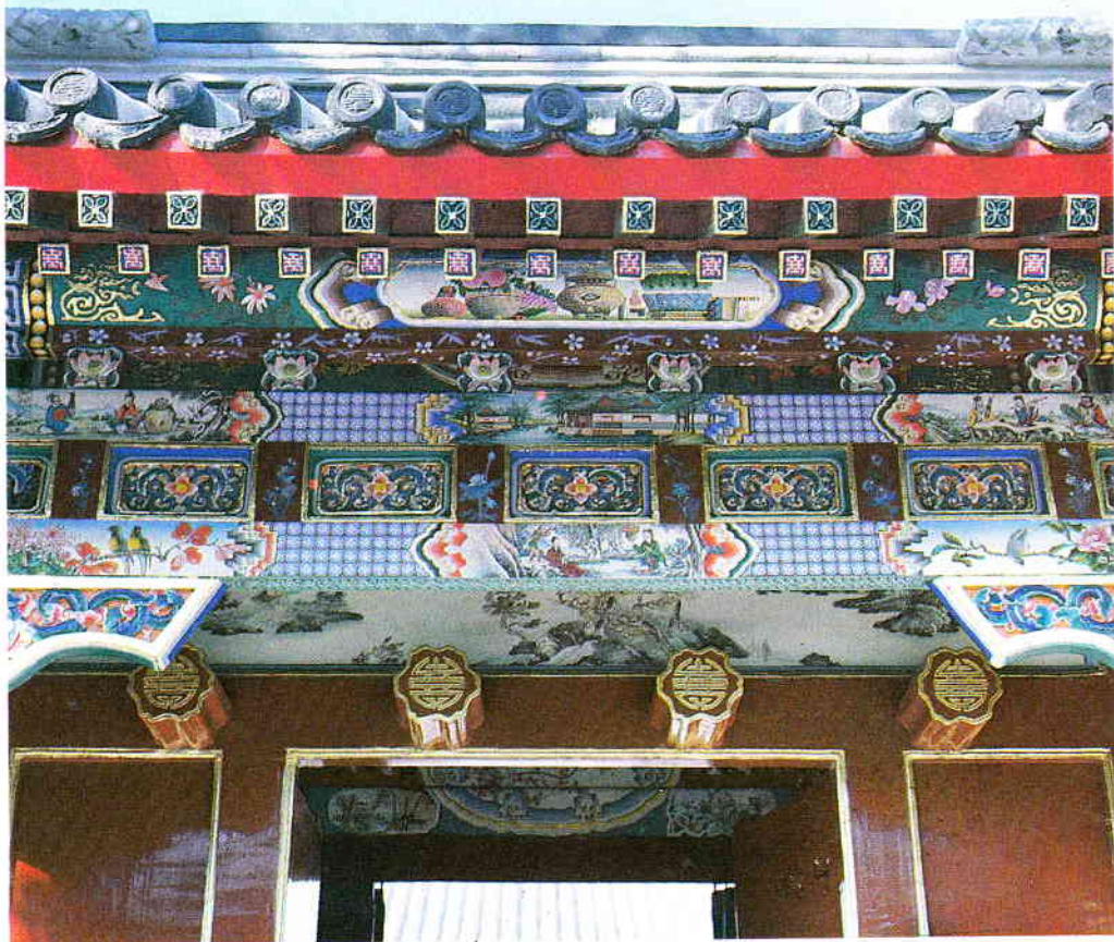
Eaves of an ancient building gleam with color after being restored.
