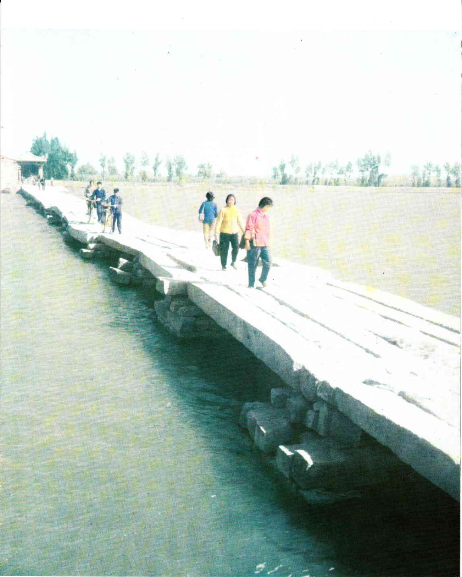
The Anping Bridge, built in the Song dynasty.
