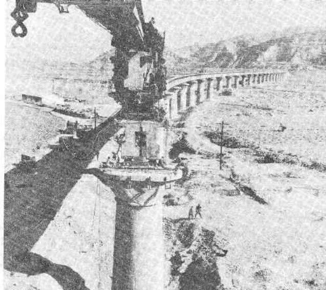
Chen Liang Bridge No. 6 across the Fenhe River.
