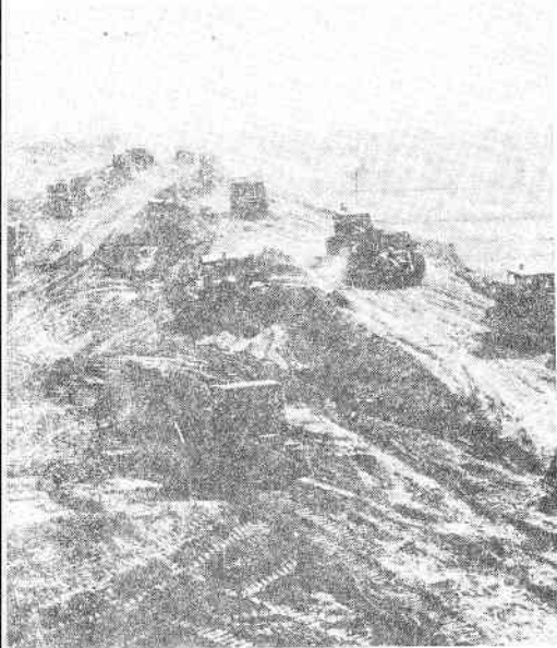
A railway under construction at the Gujiao mine.
