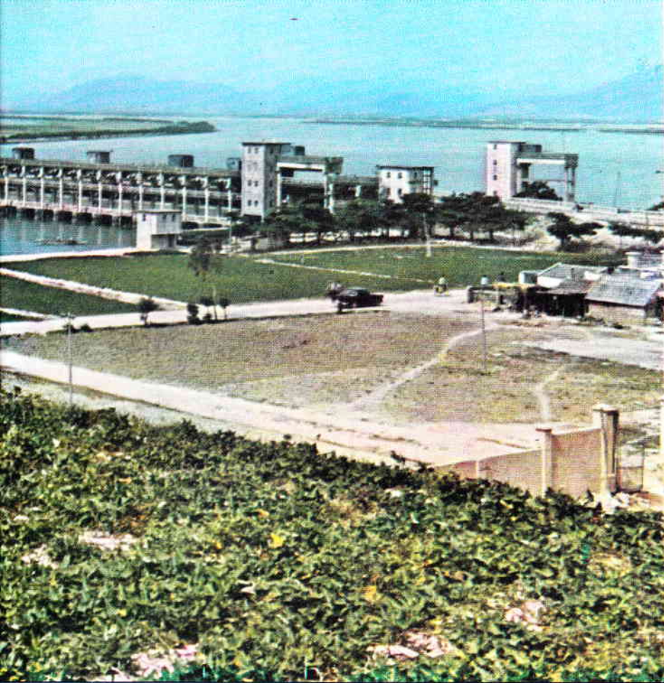
A 1,529-meter sluice to block the sea water in Chaoyang county.
