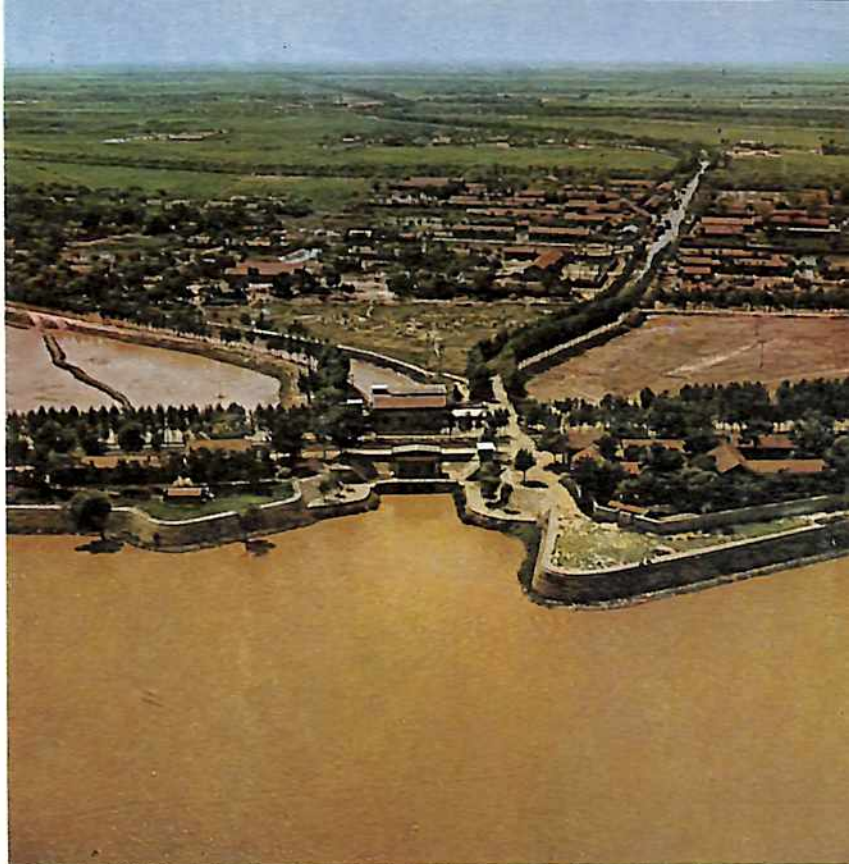
The dykes at Huayuankou on the Yellow River.
