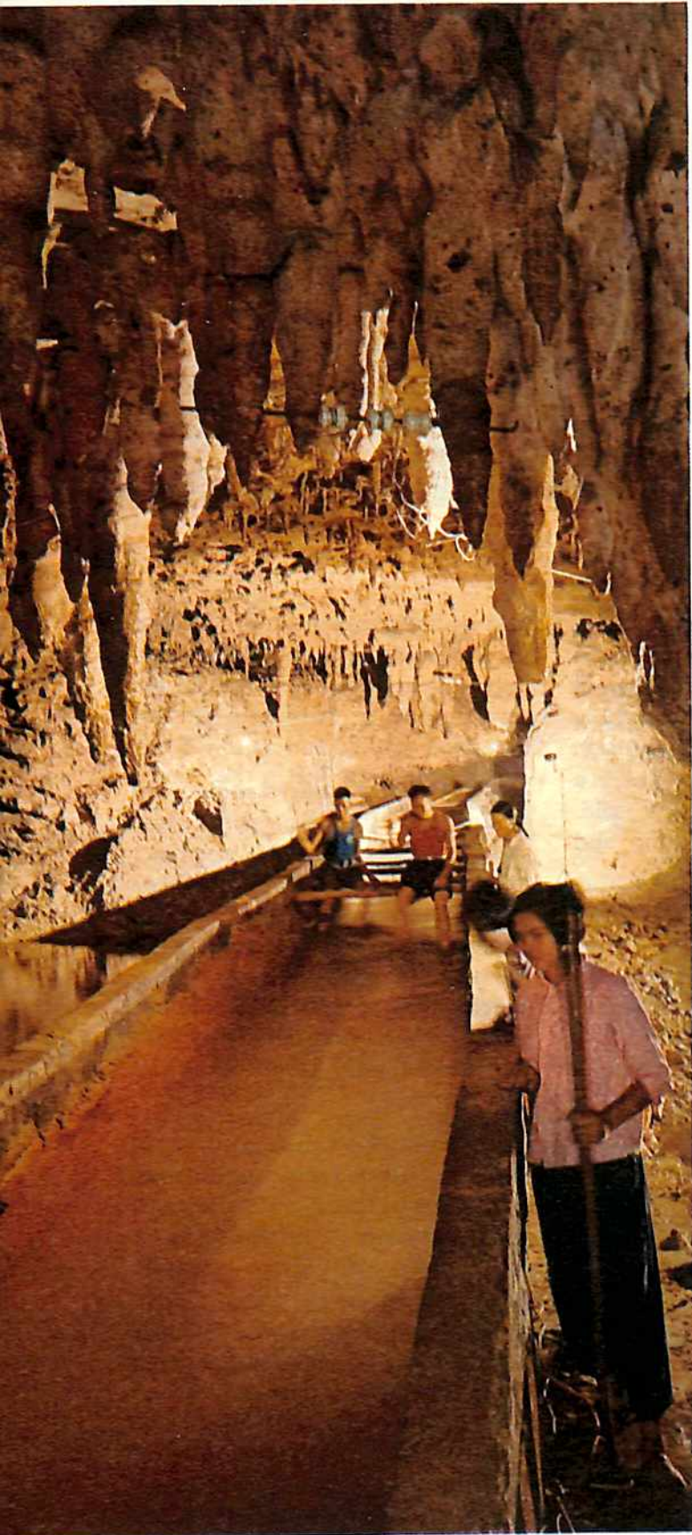
This aqueduct passes through a cave on its way to a dry mountain area.
