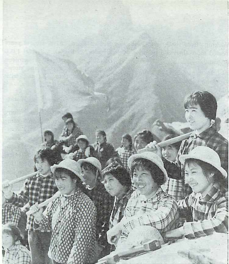
A commune all-girls' team have distinguished themselves at stone cutting, tunnel drilling and bridge building.
