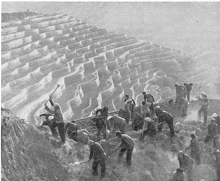
Commune members in Shensi province build terraced fields in winter.
