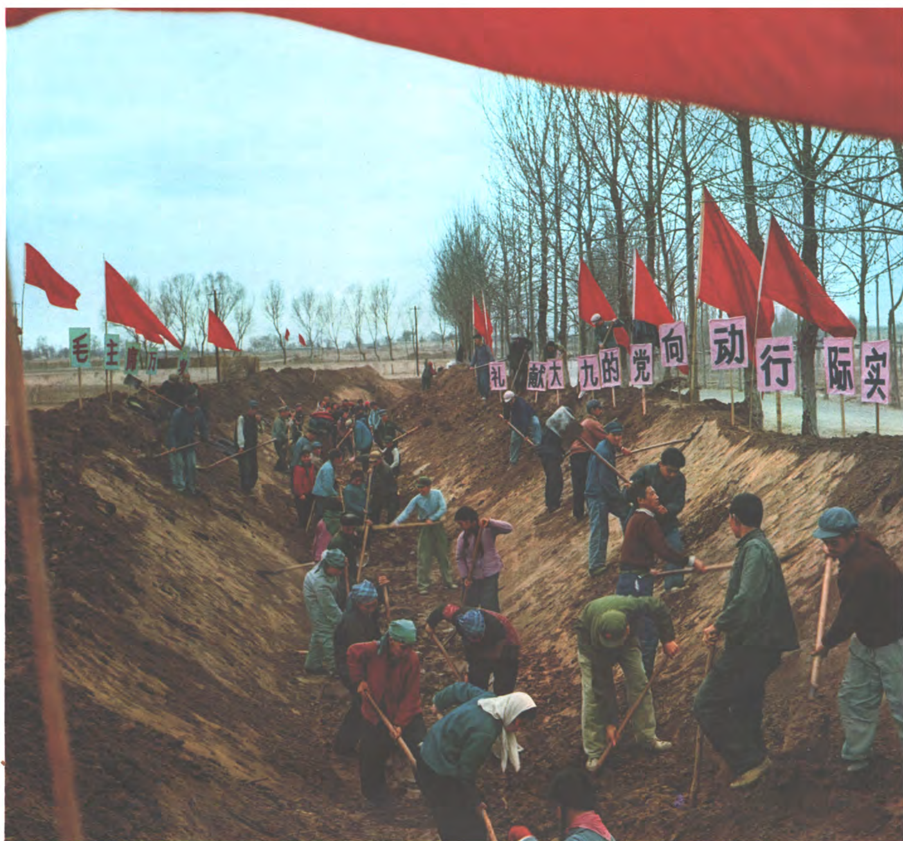
On the day after the opening of the Party's Ninth National Congress, the commune members of the Huangtukang People's Commune on the outskirts of Peking dug an irrigation channel 17 li in length, completing in one day this project on which they had planned to spend five days.
